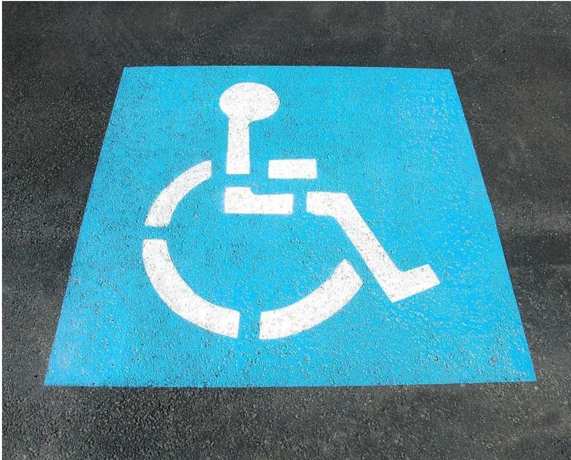
Figure 7. Designated accessible car parking space marking
